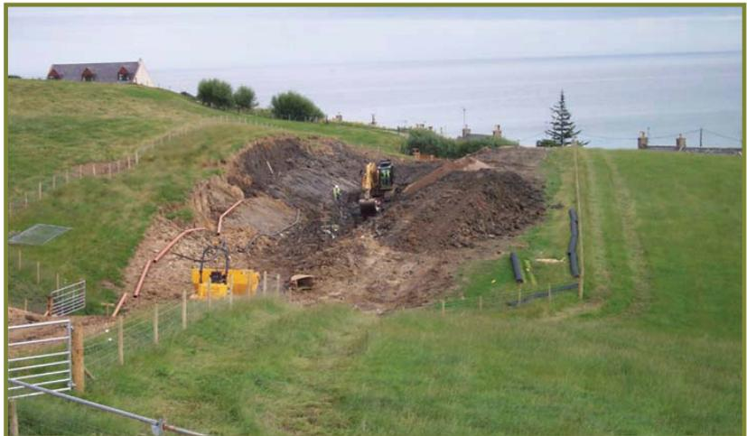
▲ At Sandend last summer, 500 metres of pipe was laid from the village uphill to a new £1 million sewer treatment plant with gravity feed back out to sea.
